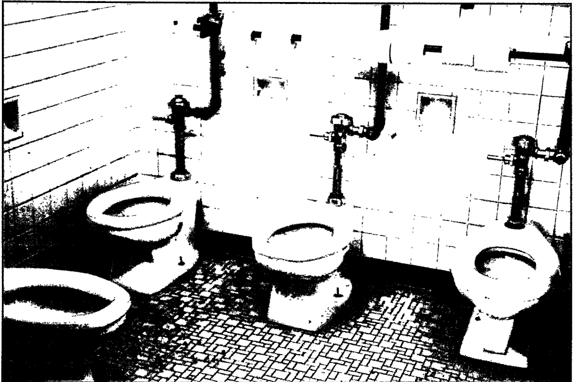
Toilet facilities at Columbus County Prison Unit
