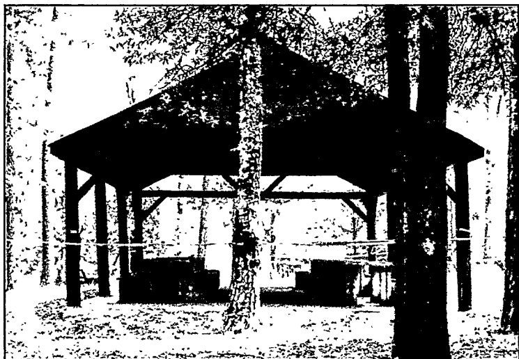
Condemned picnic shelter at Kerr Lake State Recreation Area in Vance and Warren counties
